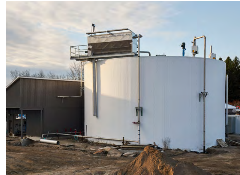
Self-Cleaning Digester at ZooShare biogas plant, Toronto, Ontario
